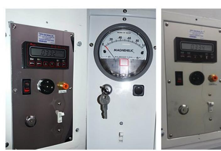
Control panel integrates control of system components in a single panel mounted at the main entry. Standard model includes ON/OFF switch & magnehelic gauge.
